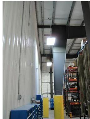
Mounting heights of the two fixtures replacing the HID are 25' high by 10 feet apart and 6 feet from the wall.
